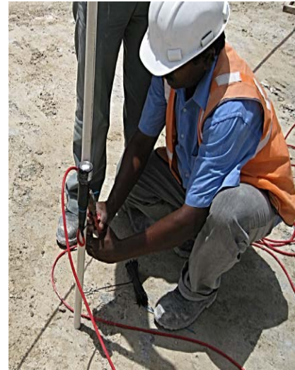
Figure 4.2 – installation by fully groutable method
